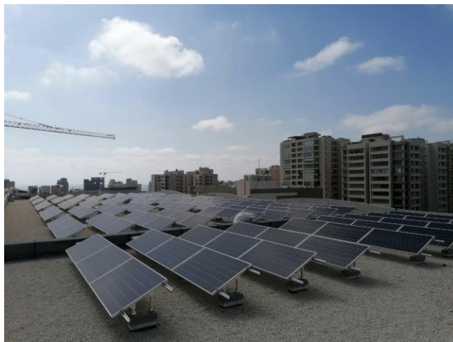
Ballasted-mount type low profile for flat roofs
