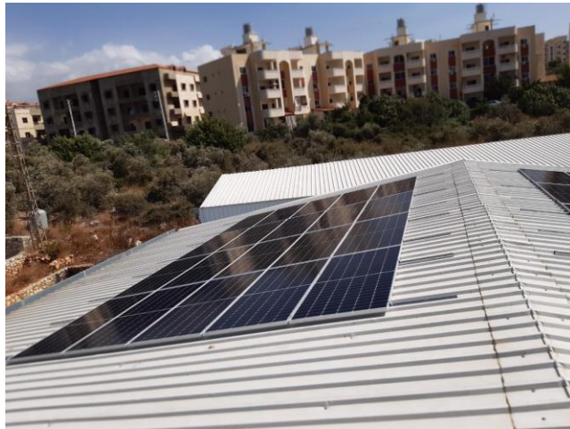
Railed mounted steel structure on pitched roof
