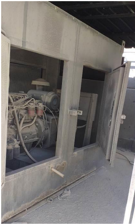
Figure 4: Zone 3 damaged generator 135kVA
